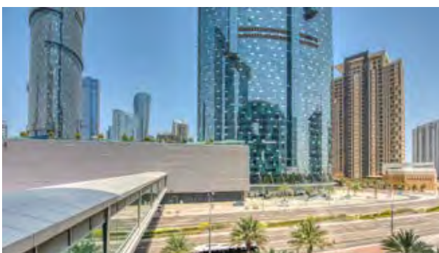
Aldar, The Arc Gate, Abu Dhabi
